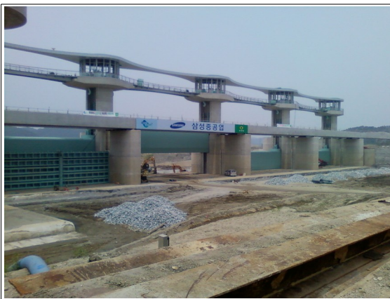
Pic 1: Floodgates under construction
