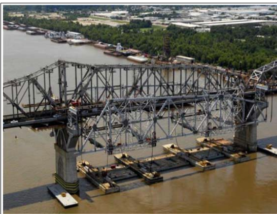
Pic 1: Huey P. Long Bridge, Mississippi River
