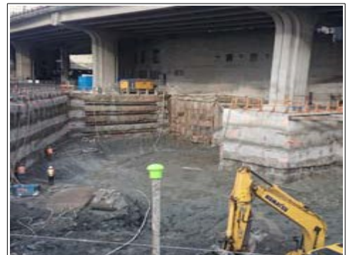
Pic 2: Construction site
