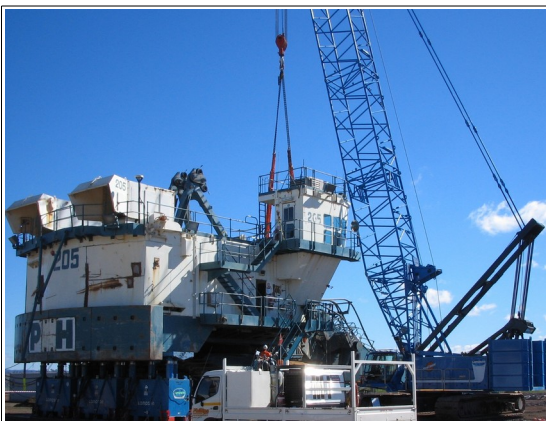
Pic 1: Lifting process
